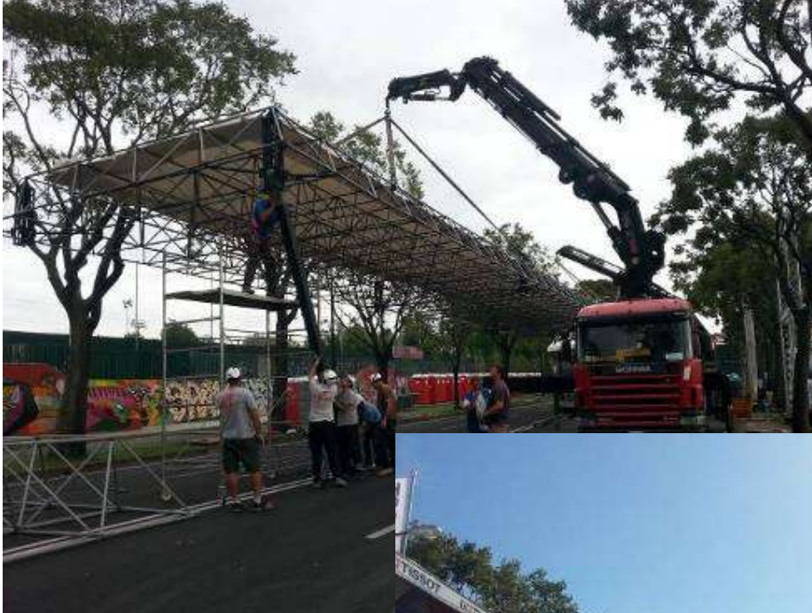
Assembly of coverings.
